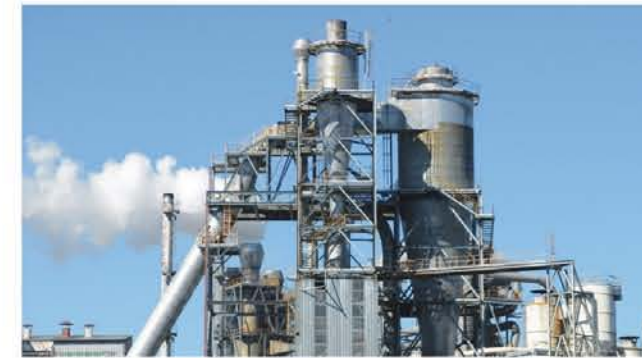
Chemical exhausted gas purification
