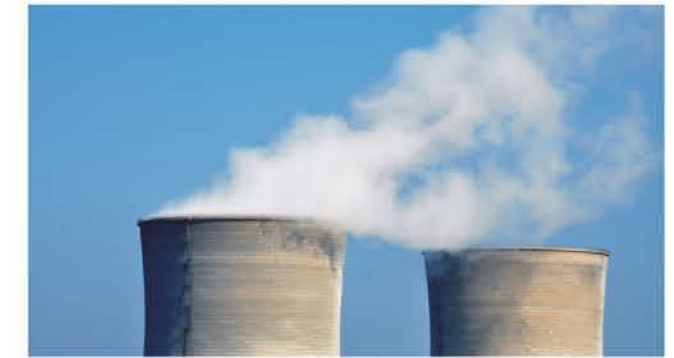
Petroleum exhausted gas purification
