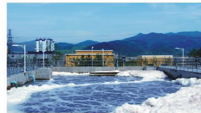
Sewage treatment purification
