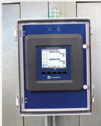
The ConsoliDator+ is fully protected from the elements by a PDA3939 NEMA 4X plastic enclosure that includes a clear front door for easy access.
