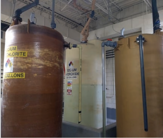
Two Hypochlorite tanks and one Hydroxide tank located inside the building
