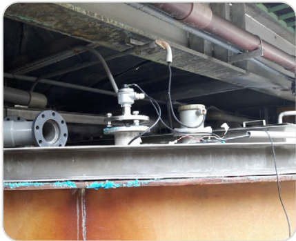
Copper sulfate storage tank
