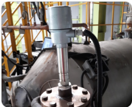
High temperature boiler
